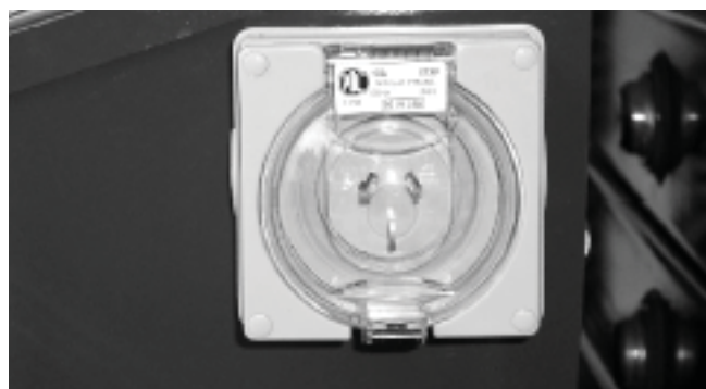
Figure 11.7 - Mains Power Connection For Charger
