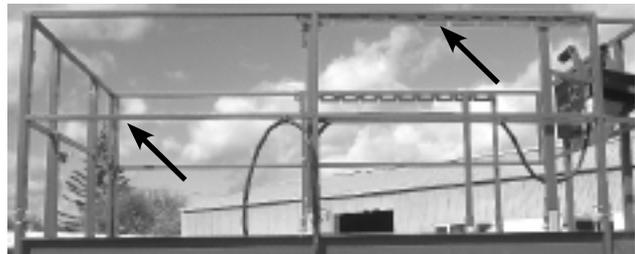
**Figure 4.5 – Fall Restraint**
