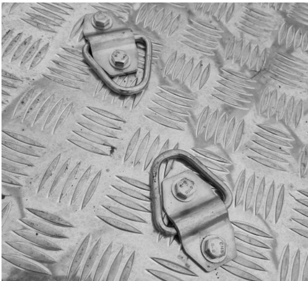
**Figure 4.15 – Fall Restraint Points**
