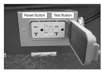
Figure 8.20 – Electrical Power Outlet
