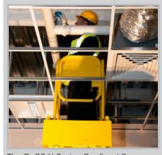
The BoSS X-Series Confined Space Guardrail has been developed to easily fit to the existing platform guardrail retainer points to allow access to restricted spaces such as the void above suspended ceilings.
